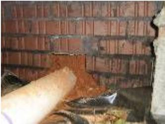
G77 It was not noted where the kitchen exhaust vent terminated, recommend checking for completion of the duct to the exterior.
