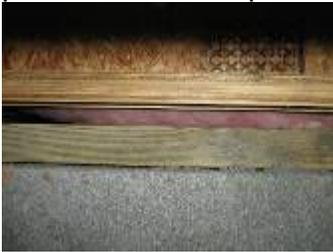
S5 Several piers have improper shimming that is already crushed in places. Shims should be at least 4 inches square and not be tapered. Tapered shims have very little bearing surface and compress. Recommend having all piers checked and corrected.
