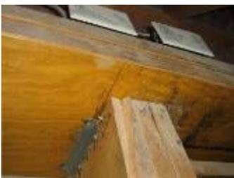
S3 Two of the deck joists have metal hangers not fully attached around the center pier.
