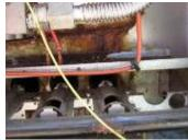
H3 The condensate line on the gas pack is missing the p-trap that is required by all manufacturers that I am aware of.
