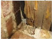
S2 The center rear has some deterioration evident at the supported ends of the band sill also. These are not fully visible and where they rest on the piers is where the rot is most likely.
